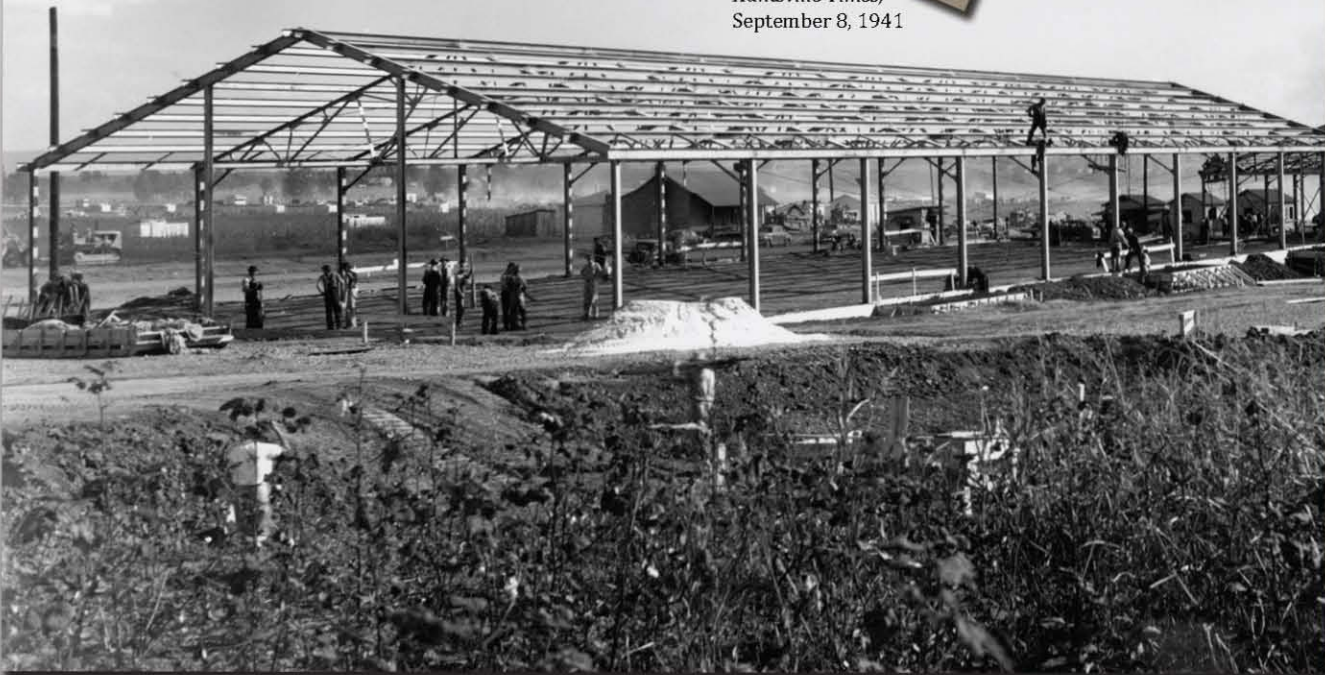
Warehouse construction, Redstone Arsenal 1941
