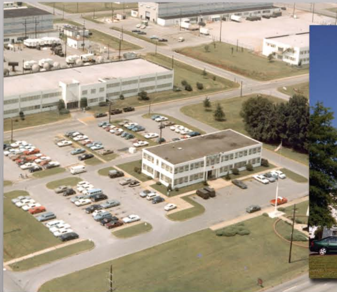
Building 3300, OMMCS (1960s)
