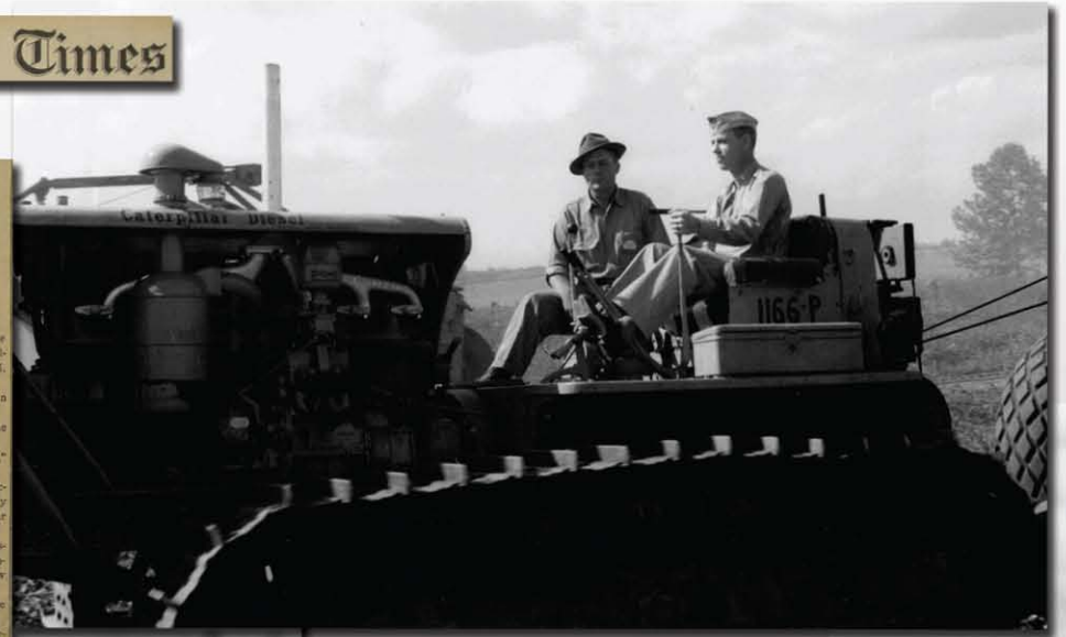
Colonel Hudson operates one of the bulldozers during the construction of Redstone Arsenal
