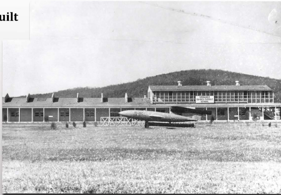
Original guided missile school building
