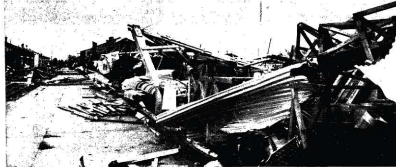
RECOGNIZE THIS PICTURE?—A pile of rubble is all that remains of three buildings on Redstone Arsenal which caught the brunt of the tornado early Monday morning. Shown here are portions of Buildings 7411, 7412 and 7402, which were completely destroyed. These buildings were located on Warehouse Road which was hardest hit by the pre-dawn twister.
