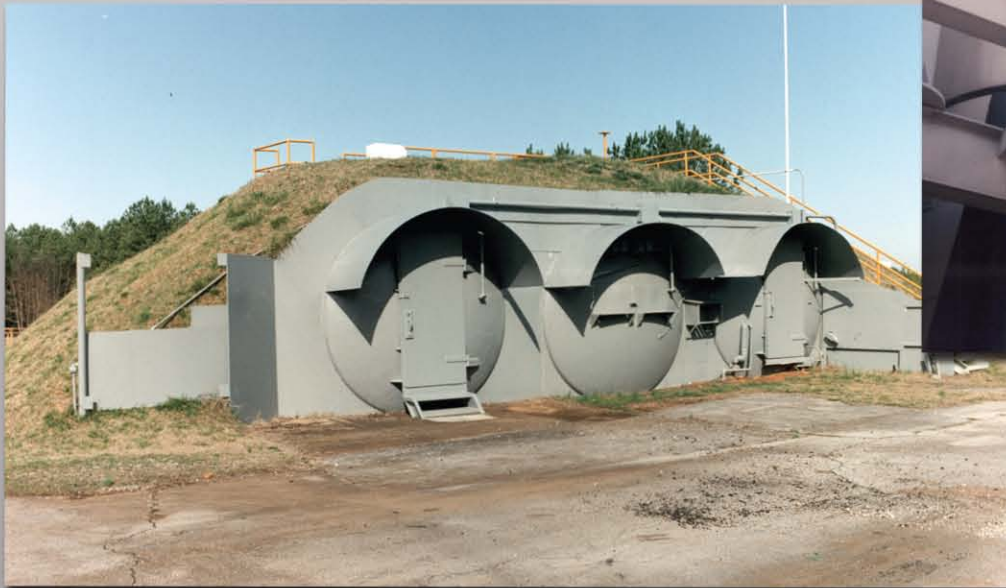
Exterior of blockhouse, 2016
