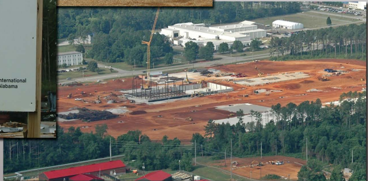
(Above) Early construction, June 2009
