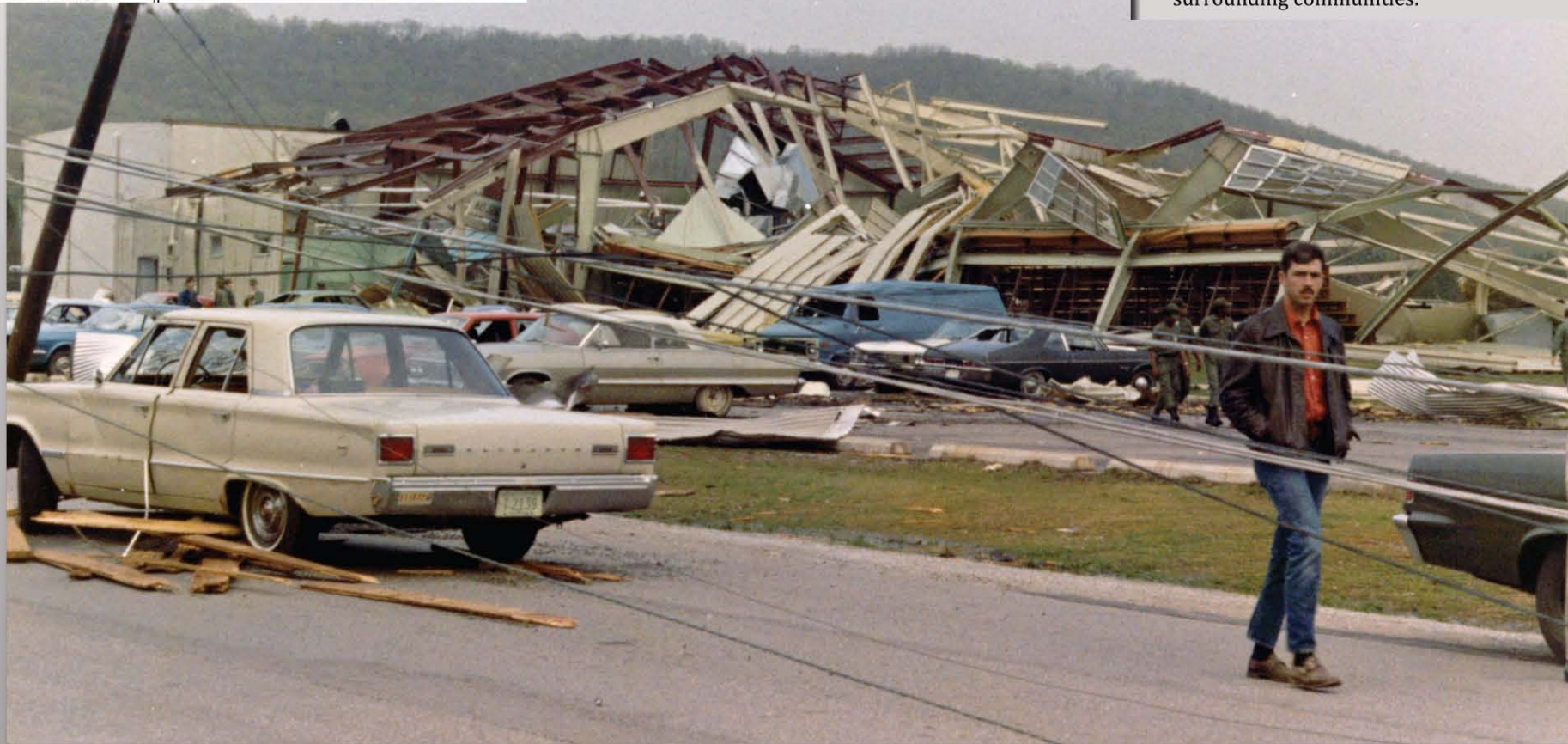
Photo of destruction taken the day after the tornado struck
