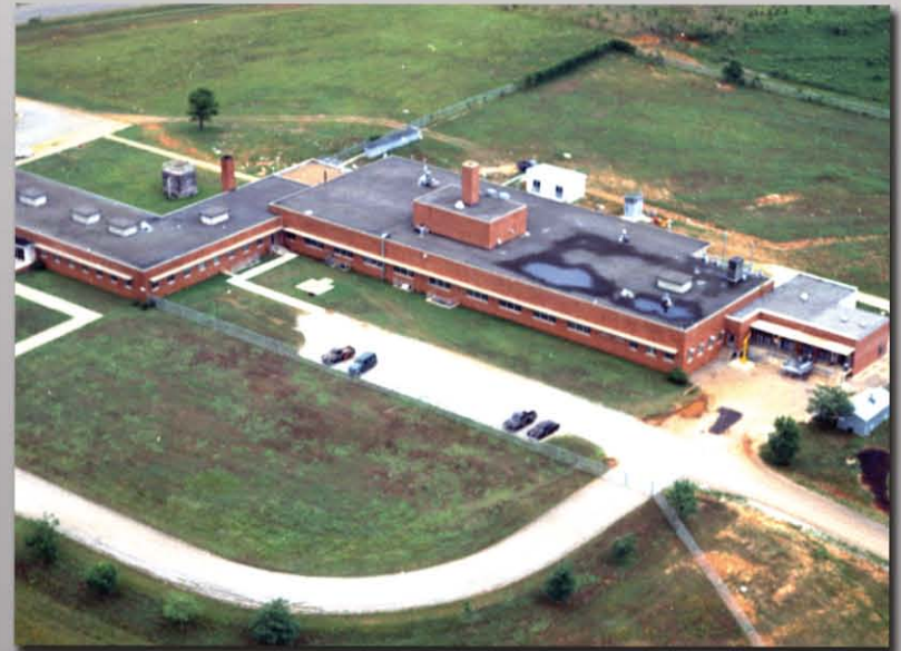
Rohm and Haas facility
